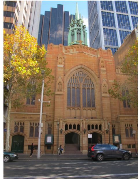
Figure 6.1 The State listed Heritage Item, St Stephen's Uniting Church, located at 197 Macquarie Street, Sydney, which adjoins the northern boundary of the subject site on Macquarie Street.
