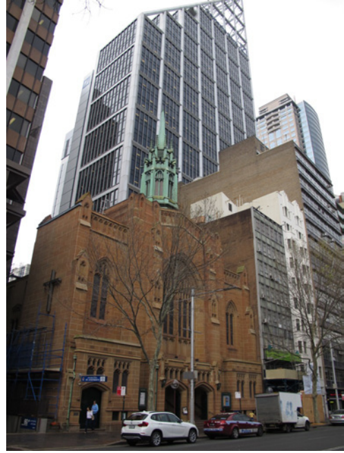
Figure 3.16 Location 6 (medium distance view): St Stephen's Church and spire as viewed from directly opposite the podium for 60 Martin Place, Sydney, on Macquarie Street.
